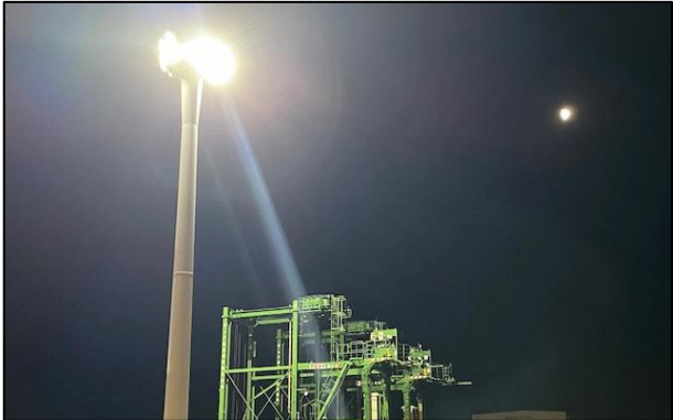
LED conversion of yard lighting
