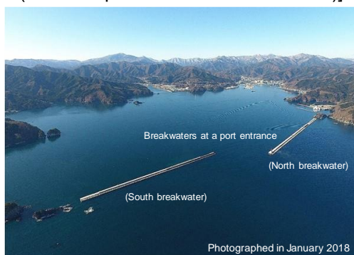
[Kamaishi Port, breakwater at the port entrance (after completion of restoration works)]
