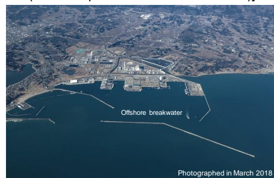
[Soma Port, offshore breakwater (after completion of restoration works)]
